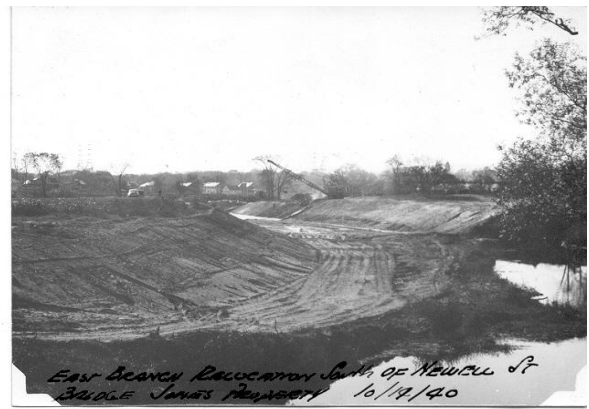
Channelization of the East Branch in Pittsfield (Source: City of Pittsfield Department of Public works & Utilities)
